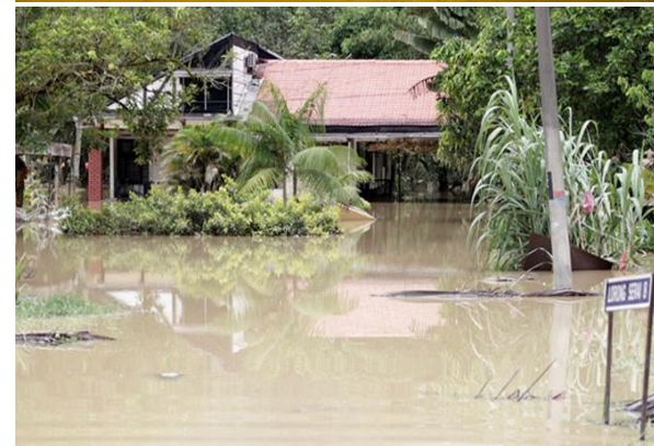
Flooding in Hulu Langat (7 March 2012)
